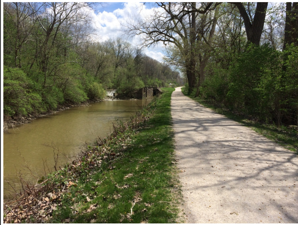
Approach to Lock 39
